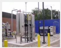
The South Monmouth Regional Sewerage Authority's combined heat and power system utilizes biogas to produce electricity and heat energy for on-site use.
