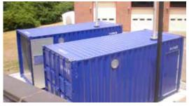
Gas is converted into power using two 140 kW internal combustion engines.
