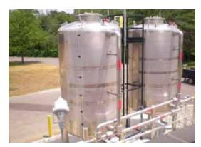
The gas conditioning equipment includes hydrogen sulfide removal through the use of H2S scrubbers.
