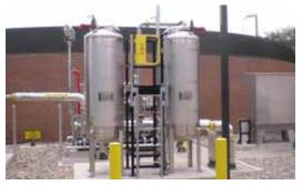
Siloxane is removed and the gas is dried and compressed.
