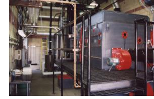
The wood waste boiler supplies heat for the kilns, and produces enough excess steam for a turbine generator to provide 150 kW of electricity for the facility.
