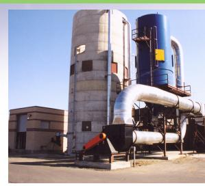
The Rex Lumber facility houses 6 wood-drying kilns that run 24 hours a day all year. By replacing a natural gas system with a woodwaste boiler to heat the kilns, the company eliminated an average annual gas bill of \$100,000. The silo in the center stores the wood waste.
