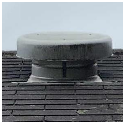
Central Supply Attic
