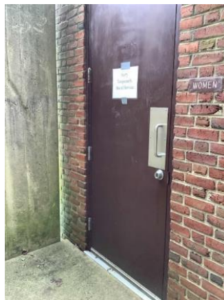
Liberty Grove Restrooms Facility Doors
