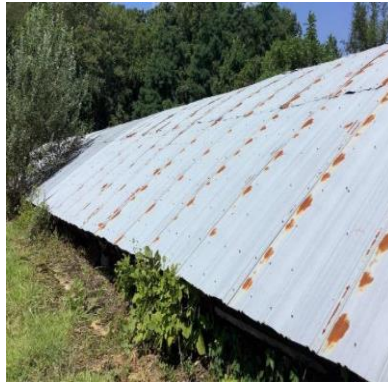
Potato Cellar Metal Roof
