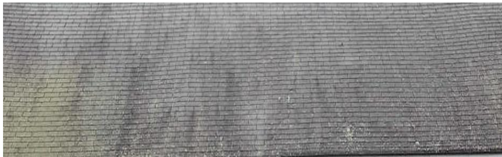
Central Supply Asphalt Shingle Roof
