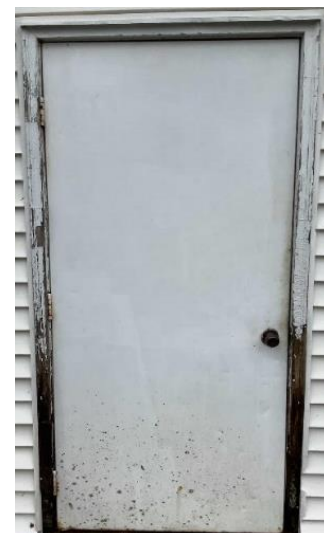
Central Supply Metal Facility Doors
