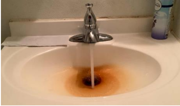
Central Supply Restroom
