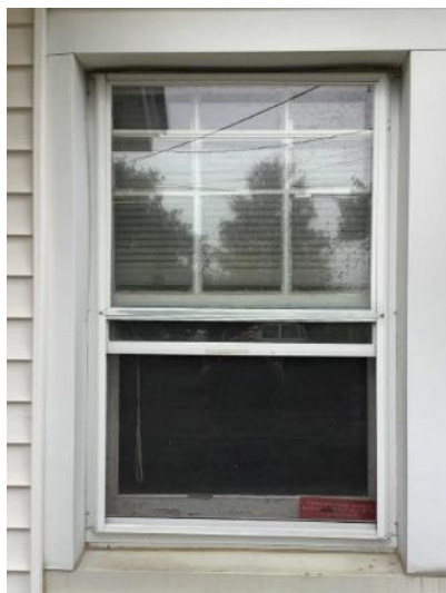
Central Supply Operable Windows w/ Storm Windows
