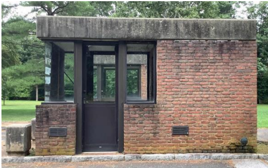
Toll Booth Envelope and Door
