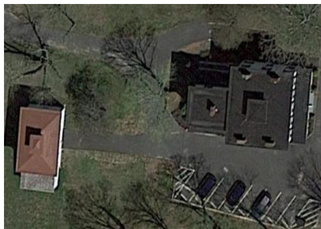
Facility Aerial View
