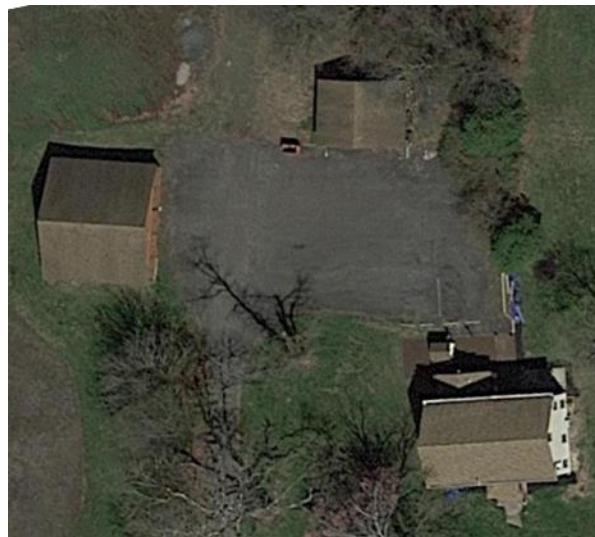
Aerial View of Facility (Bottom Right)
