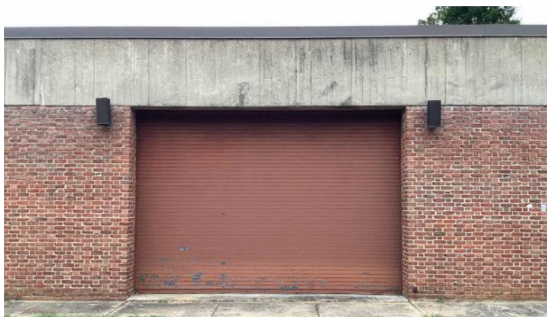
Sewer Plant Garage Door
