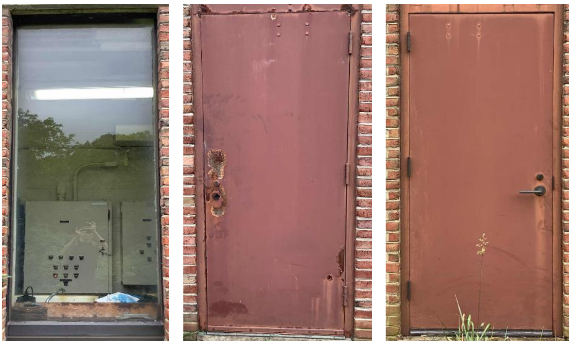
Sewer Plant Facility Windows & Doors
