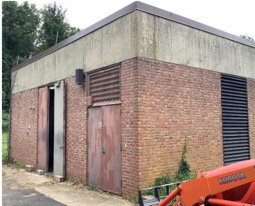
Storage Building Envelope
