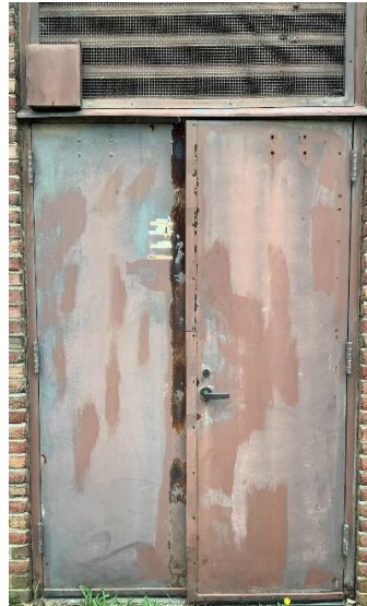
Storage Building Solid Metal Door
