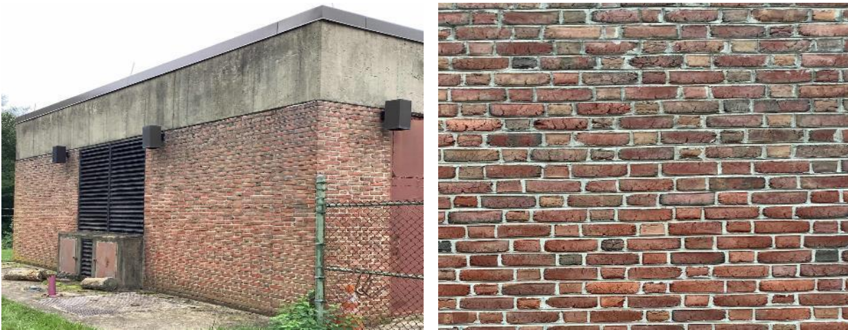
Sewer Plant Building Envelope
