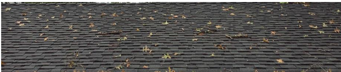
Tark House Asphalt Shingle Roof
