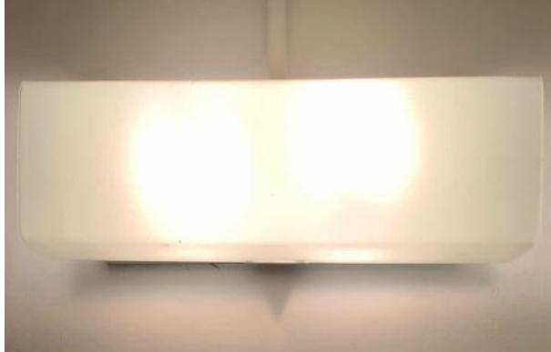
Restroom Vanity Lighting
