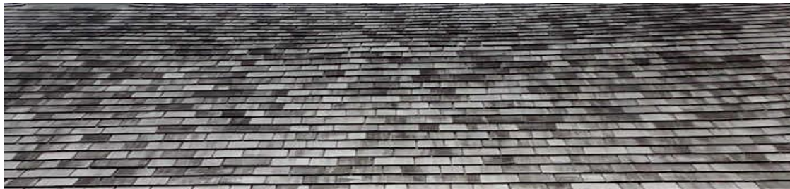
Craig House Cedar Shingle Roof
