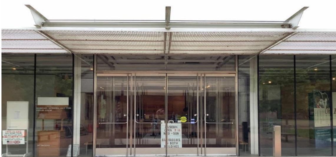
New Visitor Center Glass Doors, Floor to Ceiling Windows, and Brise Soleil
