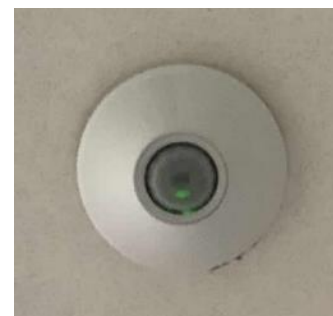
Ceiling Mounted Occupancy Sensor
