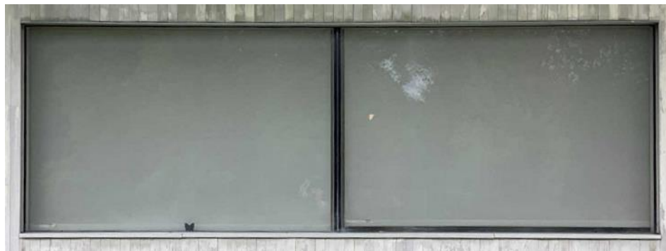
New Visitor Center Facility Windows
