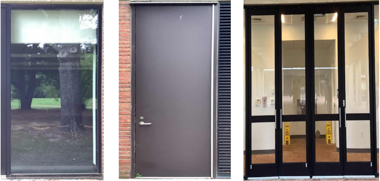
Original Visitor Center Windows & Doors
