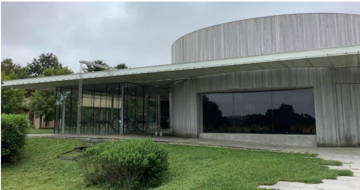
New Visitor Center Envelope and Brise Soleil
