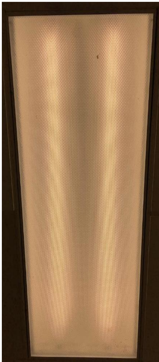
Original Visitor Center 4-Foot Linear Fluorescent T8 Tubes
