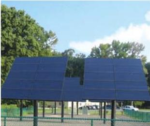
The 25 kW solar PV system generates 45 percent of the Cooperative Extension Building's electricity needs.
