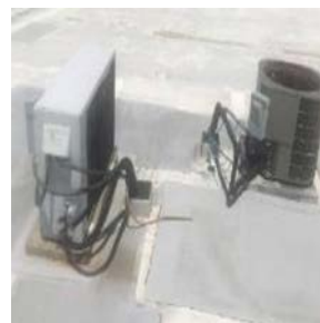
AC Condensing Unit
