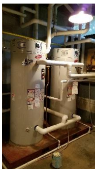
Figure 19 – High Efficiency Domestic Hot Water Heater
