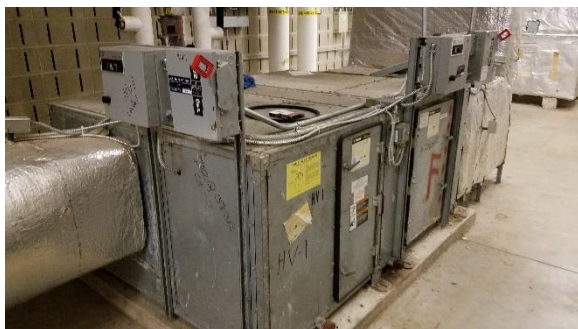
Figure 15 –AHU "HVI "
