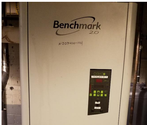
Figure 13 – Aerco high efficiency boiler
