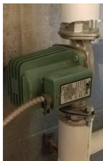
Figure 20 – Domestic Hot Water Circulator
