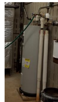
Figure 21 – Electric Domestic Hot Water Heater
