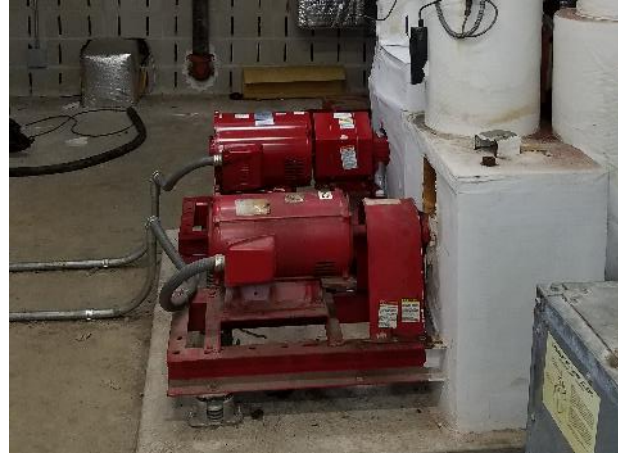
Figure 12 – 15 hp Chilled water pump
