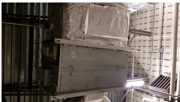
Figure 17 – Energy recovery ventilator
