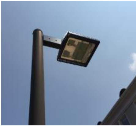
Image 7. LED Pole Mounted Fixture
