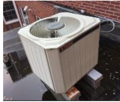
Image 10. Picture of a Split System AC Condensing Unit
