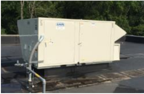
Image 9. Picture of an RTU
