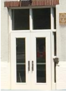
Image 3. Picture of an Exterior Door
