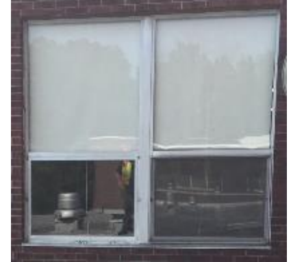
Image 5. Picture of a Window in a Newer Section of the Building
