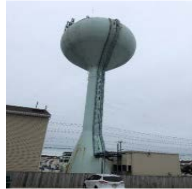
Elevated Water Tower
