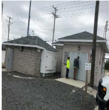
North Pump Station Building
