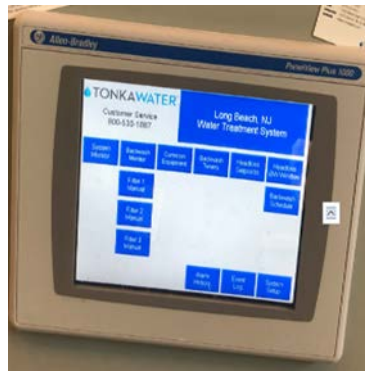
Digital Control Panel
