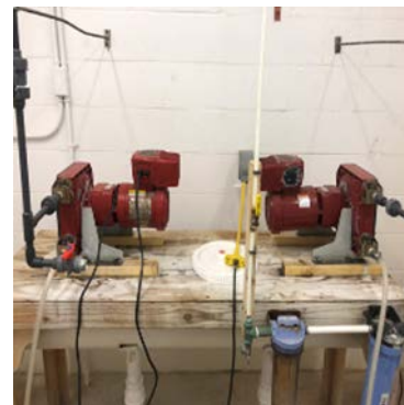
Well Pump #1 & Chlorine Pumps
