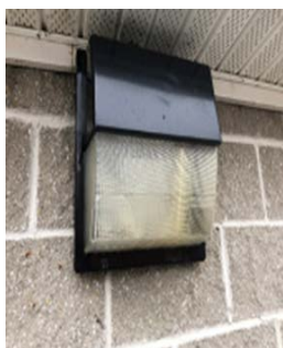
1 Typical Wall Mounted Metal Halide
