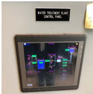
Water Plant Monitoring Panel
