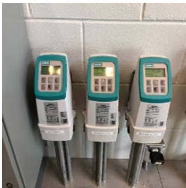
Variable Speed Drives (VFDs)
