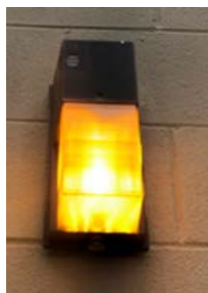
2 Typical Wall Mounted Metal Halide
