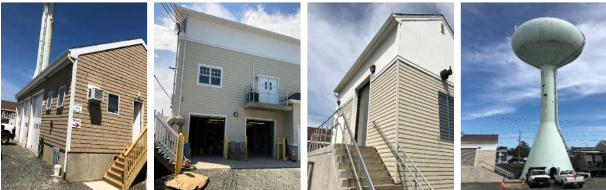
Office and Filtration Buildings
