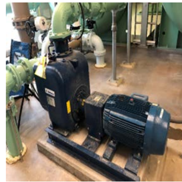
50 hp Water Pump
