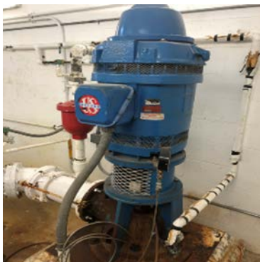
Well Pump #1 & Chlorine Pumps
