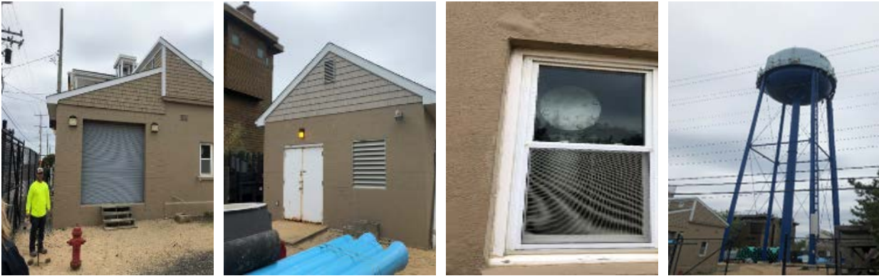
Generator-Chlorine & Well Buildings
