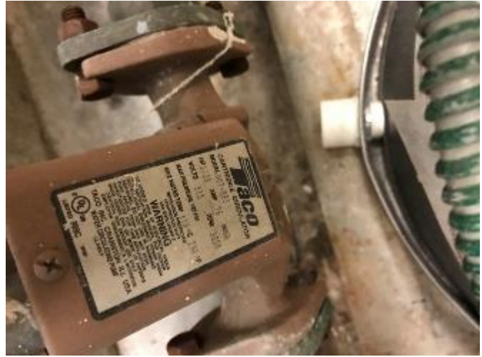
DHW Circulation Pump
