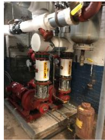
Hot Water Heating Pumps
