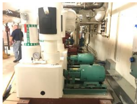
Chilled Water Pumps
