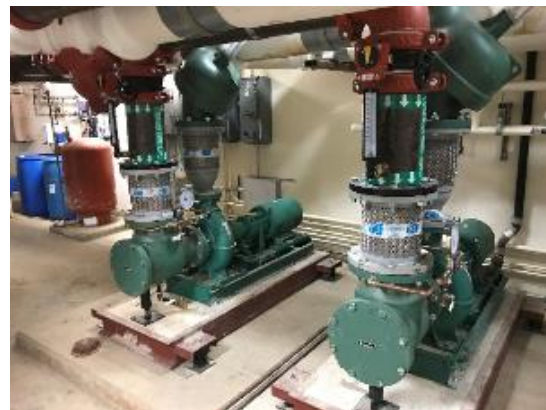
Condenser Water Pumps
