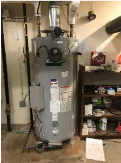
Gas DHW Heater
