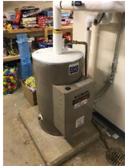
Electric DHW Heater
