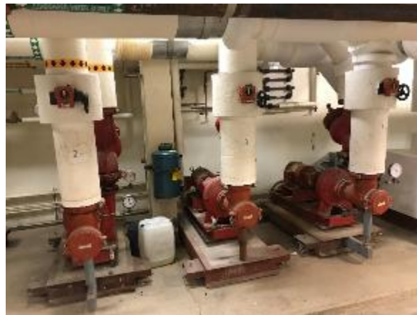
Hot Water Pumps
