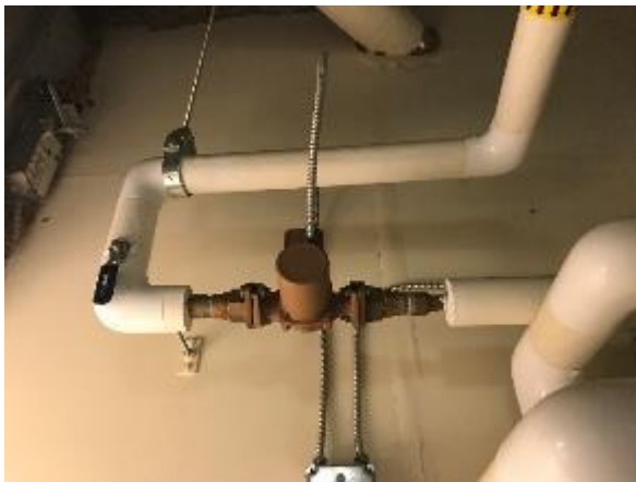
DHW Circulation Pump
