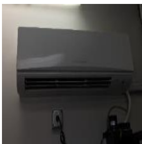
Server Room AC Evaporator Unit
