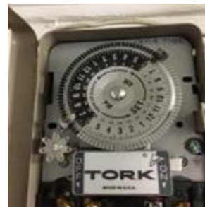
Exterior Lighting Timeclock
