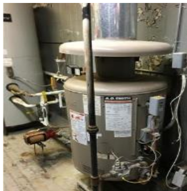
DHW Water Heater
