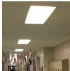
Recessed Hallway Fixtures
