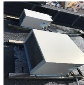
Walk-In Units Condenser Units
