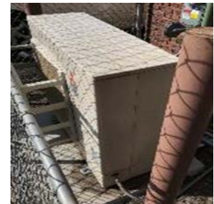
Split System AC Condensing Unit
