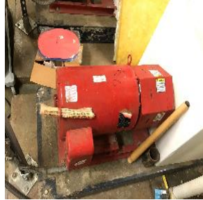
Chilled Water Pump (P-6)
