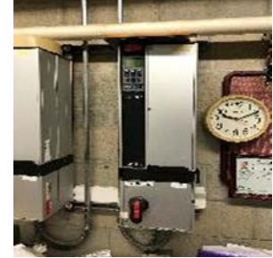
Chilled Water Pump VFD (P-6)
