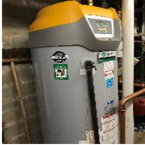
Water Heaters (DHW)
