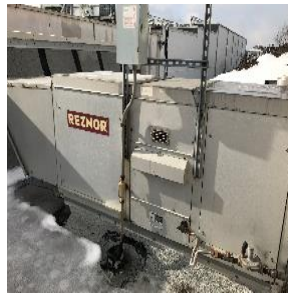
MAU on roof
