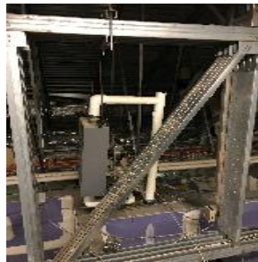
Unit Heater in the Attic
