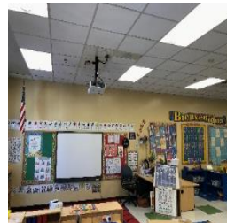
T8 Fixtures (Classroom)
