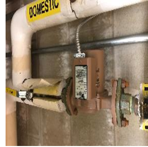
DHW- Recirculation Pump
