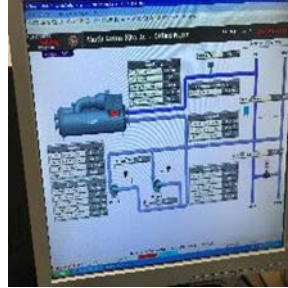
Chiller and CHW Pumps (EMS)
