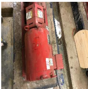
Heating Hot Water Pump (P-1)
