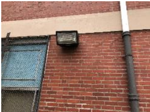
Outdoor Wall-mounted Fixtures
