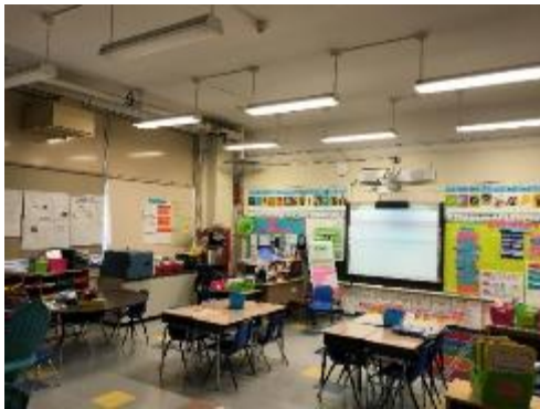
Ceiling-mounted T8 Fixtures
