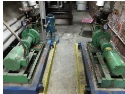
Hot Water Pumps
