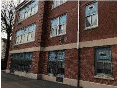
Brick Façade and Windows
