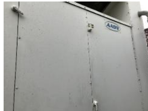
Gym Packaged Units
