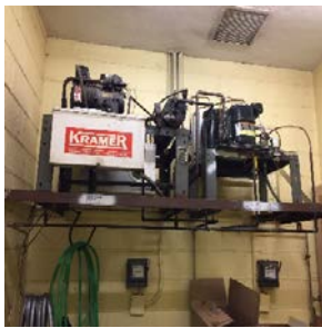
Walk-in Cooler/Freezer Compressors
