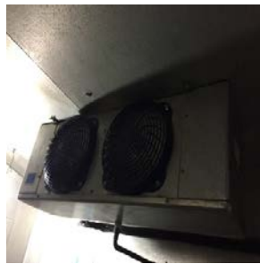
Walk-in Cooler/Freezer Evaporators
