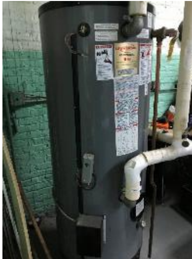
Domestic Hot Water (DHW) Heater
