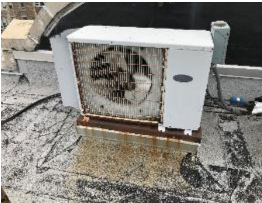
Split AC Unit
