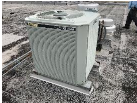
Split AC Unit
