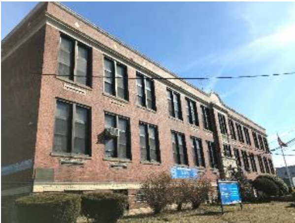
Building Façade and Windows
