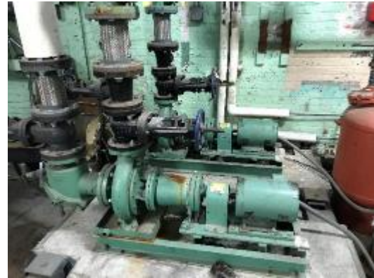
Hot Water Pumps
