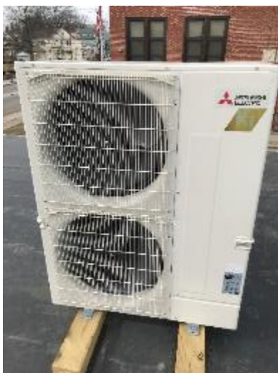
Split AC Unit
