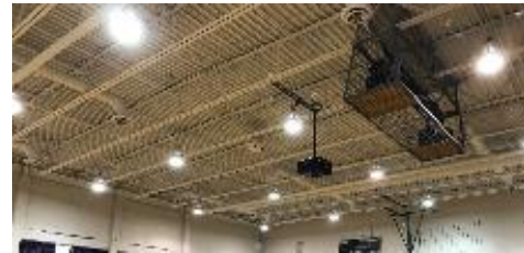
Gym High Bay Fixtures
