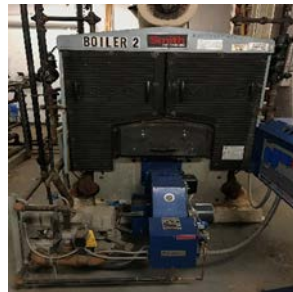
Old Wing Boiler
