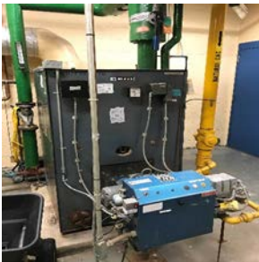
New Wing Boiler
