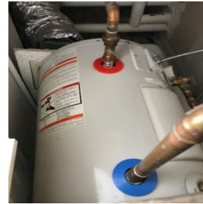
Electric Water Heater
