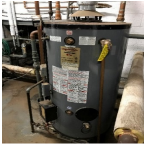
Gas Water Heater
