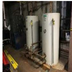
Indirect DHW Storage Tanks
