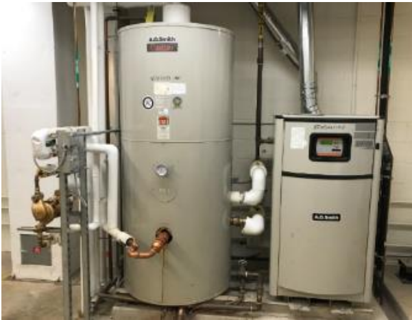
Water Heater and Storage Tank
