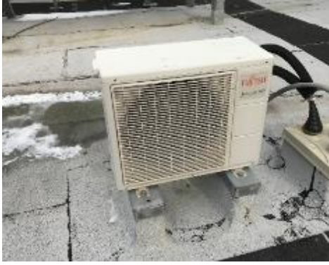
Split System Air-Source Heat Pump
