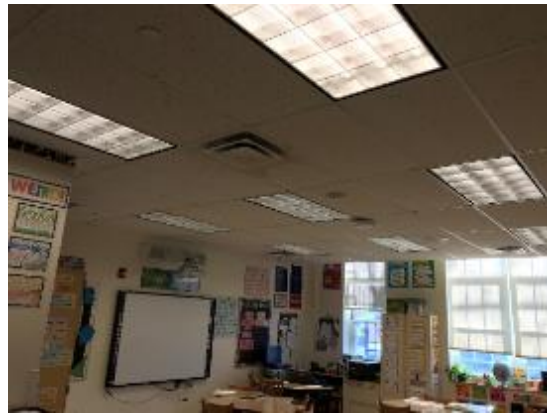
Surface Mount Linear Fluorescent T8 Fixtures
