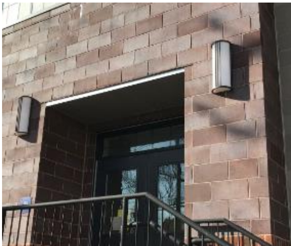
Exterior Wall Pack CFL Fixtures
