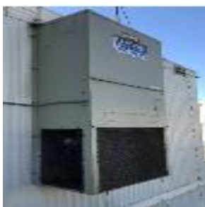
Wall-Mounted PTAC Unit
