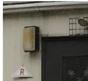
TCU Exterior Wallpack
