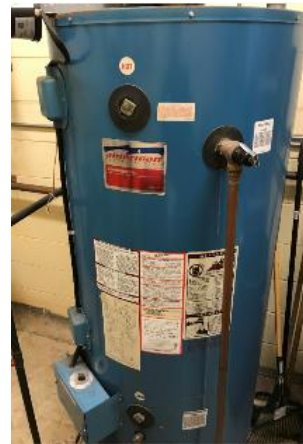
New Wing DHW Heater
