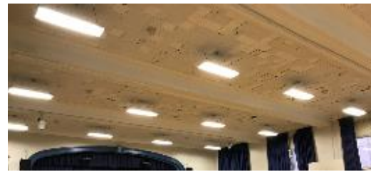
Gym Lighting Fixtures
