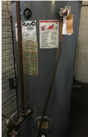
Old Wing DHW Heater
