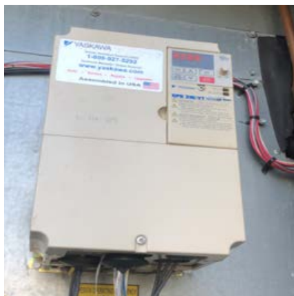
Supply & Return Fans Variable Speed Drives
