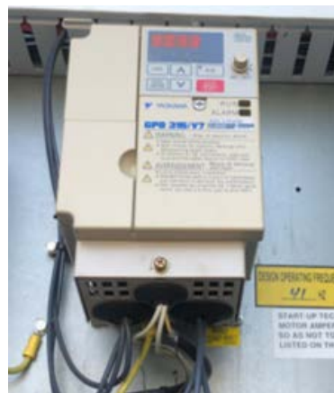
Supply & Return Fans Variable Speed Drives
