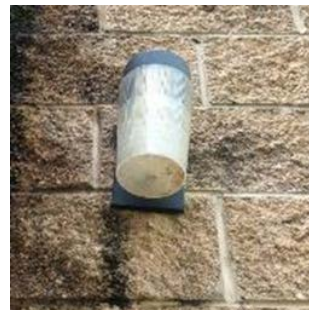
Exterior Wall pack Fixture
