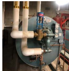
DHW Heat Exchanger
