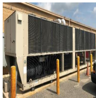
Air-Cooled Screw Chiller
