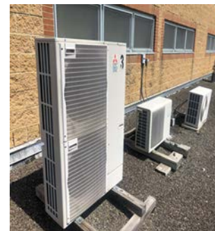
Split System AC Condensing Units
