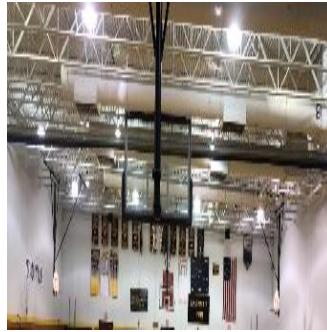
Gym Lighting Fixtures
