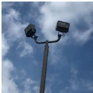
Exterior Pole Mounted Fixtures
