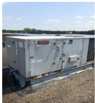
Rooftop Packaged Unit
