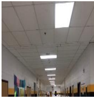
Hallway Lighting Fixtures
