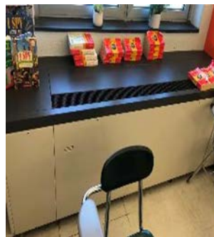
Classroom Unit Ventilator
