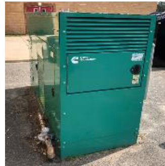
Gas Fired Back-Up Generator
