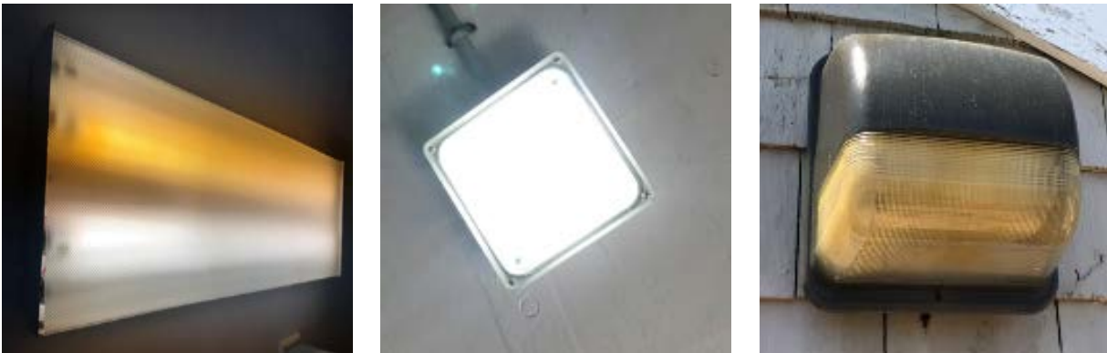
Linear Fluorescent T12, LED, and HPS Fixtures
