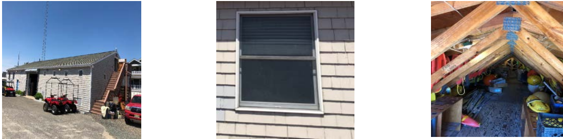
Beach Patrol Building Walls, Window and Attic Floor
