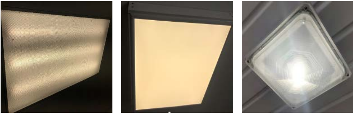
Interior T8 and LED Fixtures
