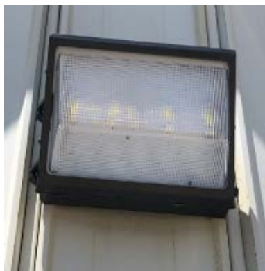
250-Watt Metal Halide and LED Wall Mounted Fixtures
