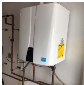
Tankless Gas-Fired Water Heaters at Holgate Restrooms and Bayview Park
