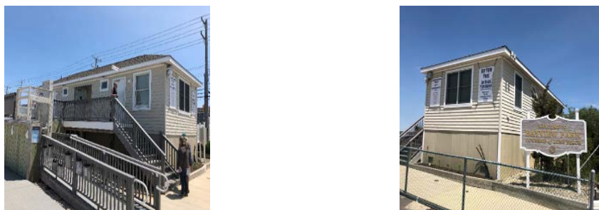
Bayview Park Building
