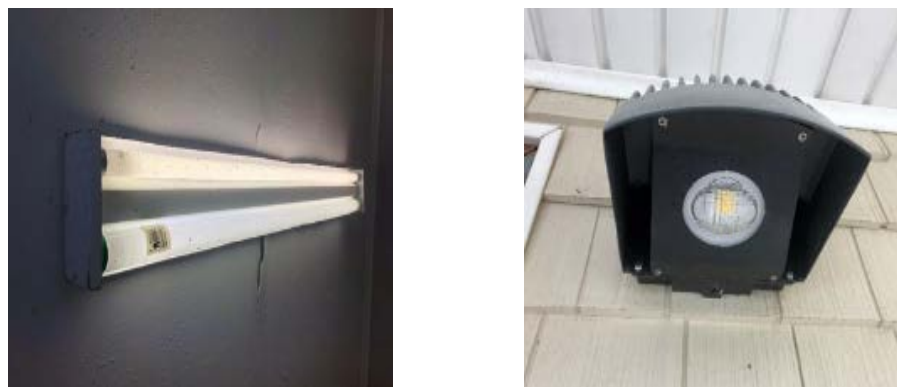
Interior T12, and Exterior LED Fixtures
