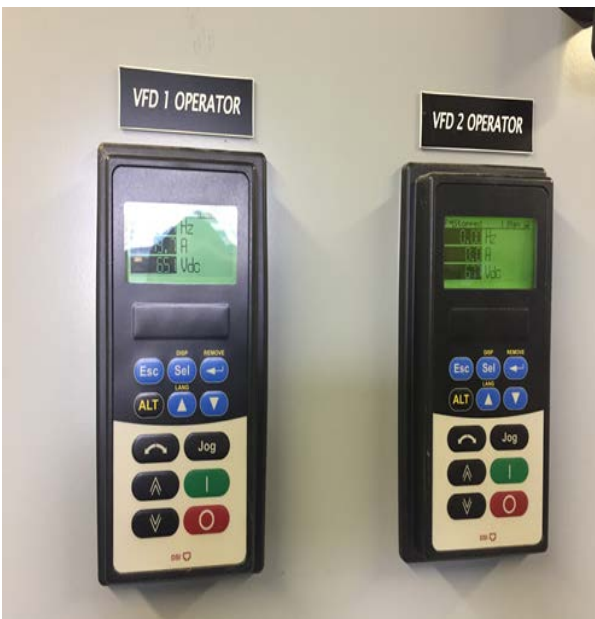
Image 5: Hydraulic Grinder Pump, Variable Frequency Drive Controls & Exhaust Fan
