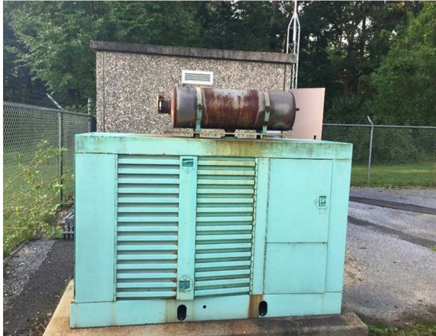
Image 1: Building Exterior View
