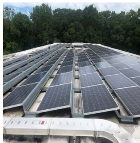
Rooftop Solar Array
