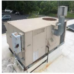
Rooftop Packaged Unit
