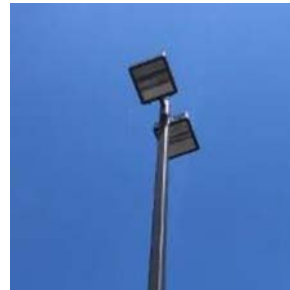
Image 11. Pole Mounted Fixtures
