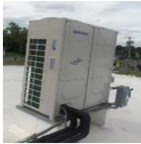
VRF Condensing Unit
