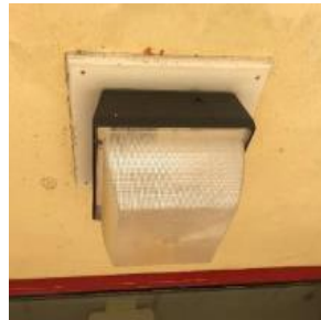
Image 10. Surface Mounted Exterior Fixture
