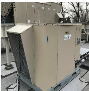
Rooftop Package AC Unit
