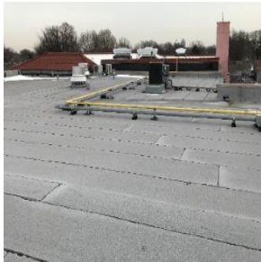
Site's Roof Cover with Black Membrane
