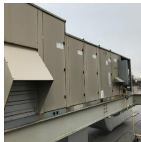
13 ton - Energy Recovery Unit
