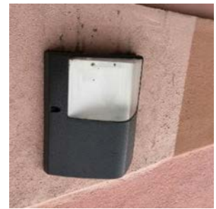
Exterior Wall Fixture
