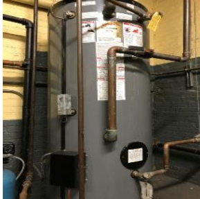
Domestic Hot Water (DHW) Heater
