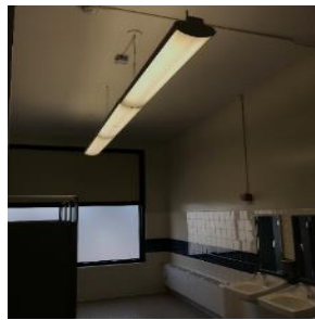
Restroom's Linear Fluorescent Fixture
