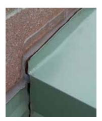
Gutters were also found to be either full of organic debris or other objects such as tennis balls or stones. Some gutters' seams were found to be leaking and in other areas downspouts were found to be disconnected from the gutters.
