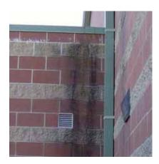
The same cap flashing seam leakage issue can also be attributed to signs of water seepage behind installed gutters. Other caulked end-seams were also found to be failing.
