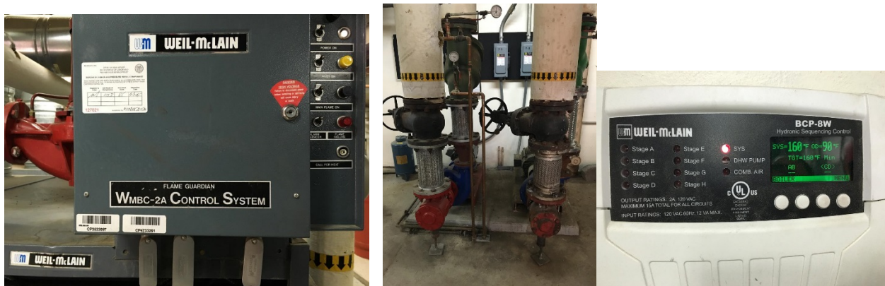
Image 4: Main Boilers and How Water Pumps
