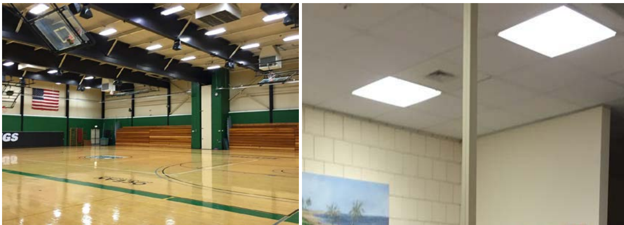
Image 2: Interior Lighting Fixtures
