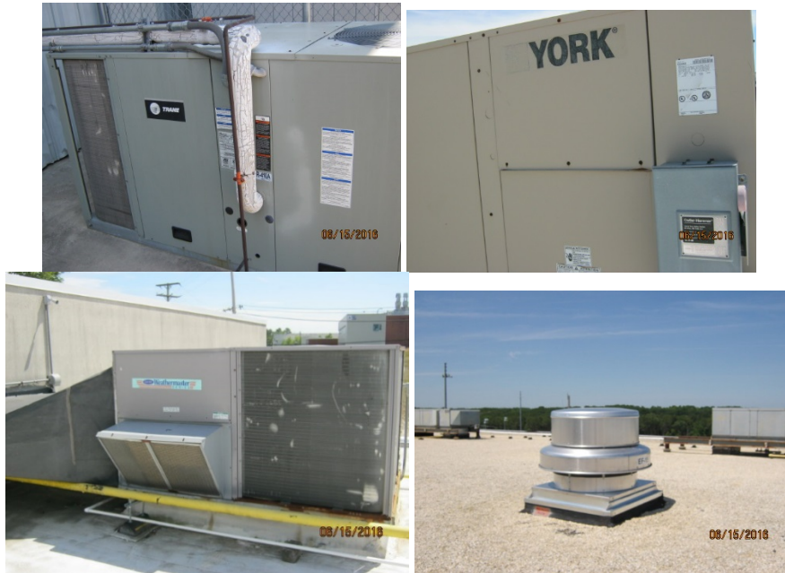
Image 5: Rooftop Units and Exhaust Fans
