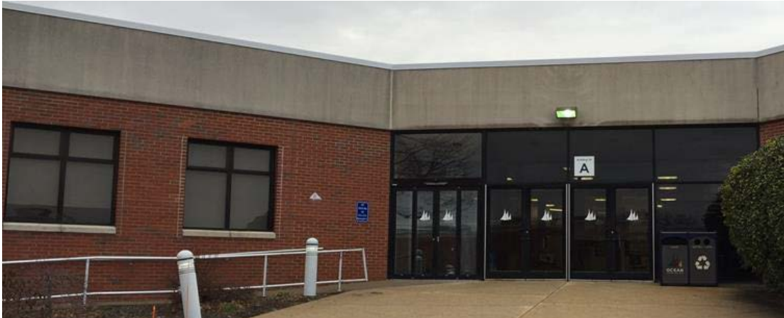
Image 1: Building Front Entrance
