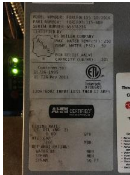
Image 6 – Boiler nameplate
