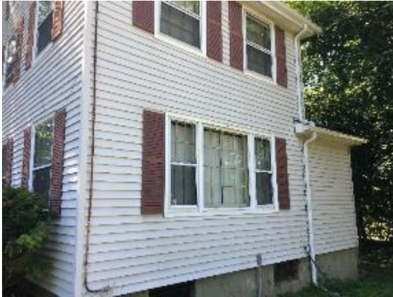
Image 1 – Wood framed windows w/storm windows
