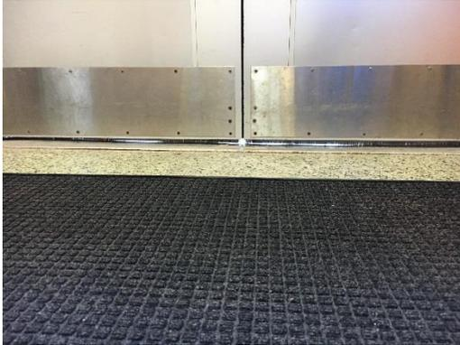
*Exterior Door with Worn Weather-Stripping*
