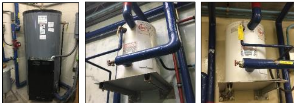
Image 5: Domestic Water Heating
