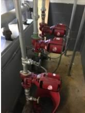
Hot Water Pumps
