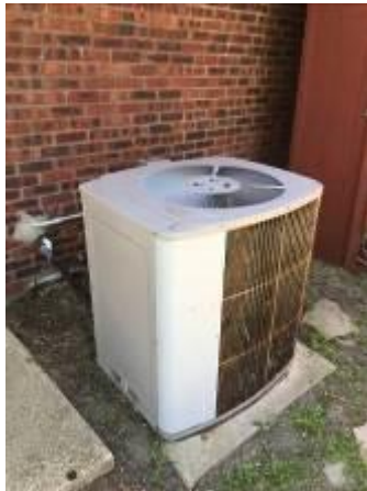
Split System Condenser
