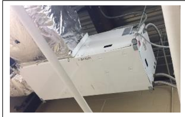
Figure 9 – Air Conditioning (DX) Systems
