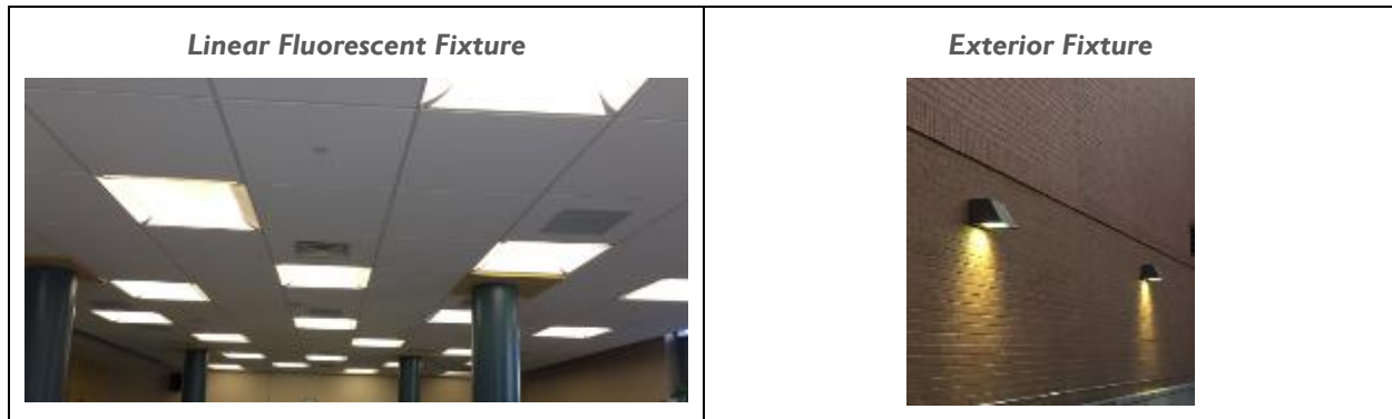
Figure 7 - Building Lighting Systems
