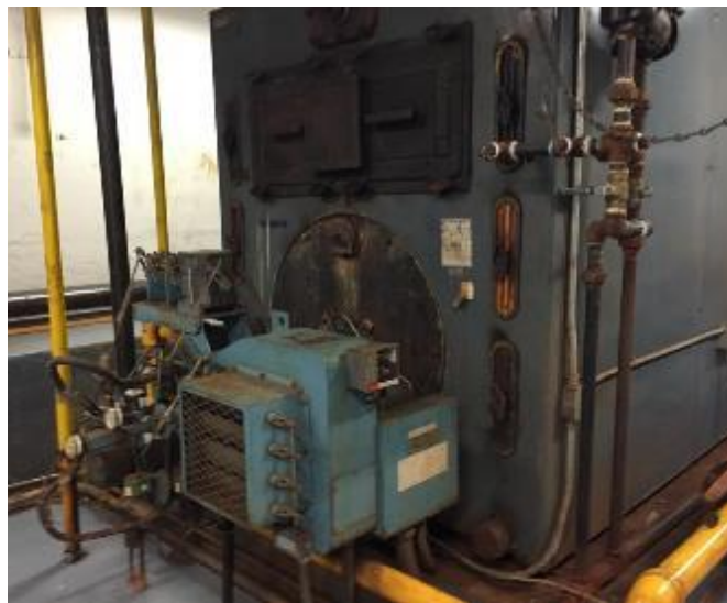
Image 3: HVAC at Buzz Aldrin Middle School
