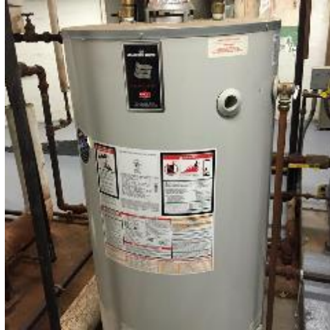
Image 4: Domestic Hot Water at Buzz Aldrin Middle School
