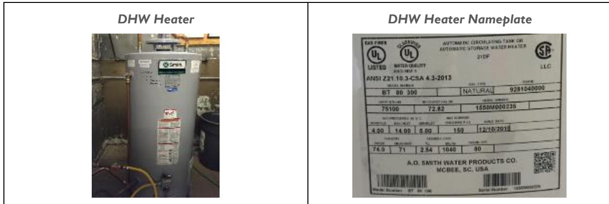
Figure 12 – Domestic Hot Water System
