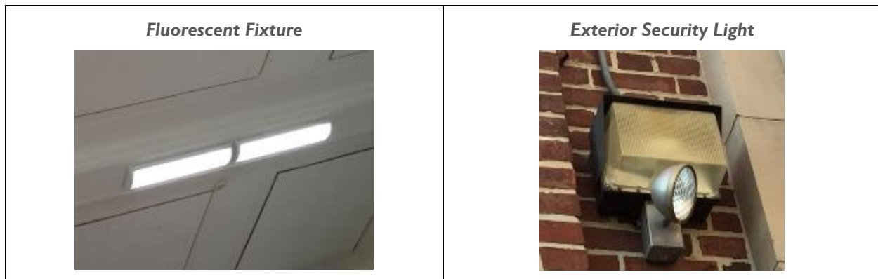
Figure 9 - Building Lighting Systems
