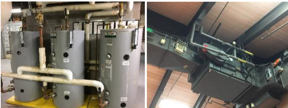
Image 3 DHW storage tanks and Gym Air Handling Unit
