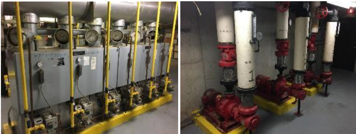
Image 2 Boilers and Circulating motors
