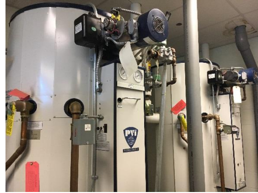
Athletics Area Storage Tank Water Heaters
