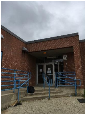
Under Canopy Fixture – On during Daytime
