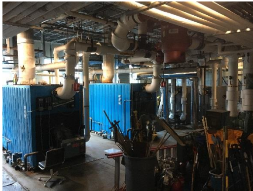
Non-Condensing Hot Water Boilers
