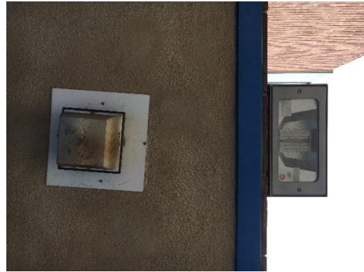
Under Canopy & Wall Pack Fixtures
