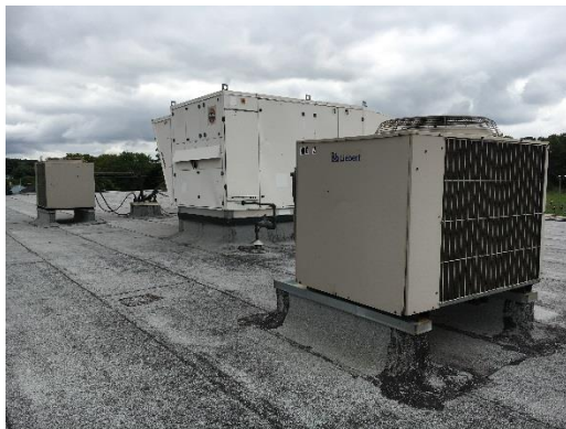
Split AC Systems – Outdoor Condensing Units
