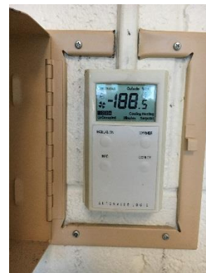
Broken Thermostat
