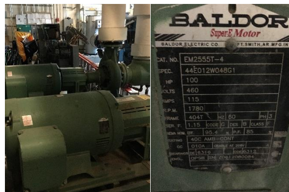
Hot Water Pumps and Motor Nameplate
