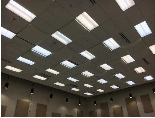
Band Room Lighting
