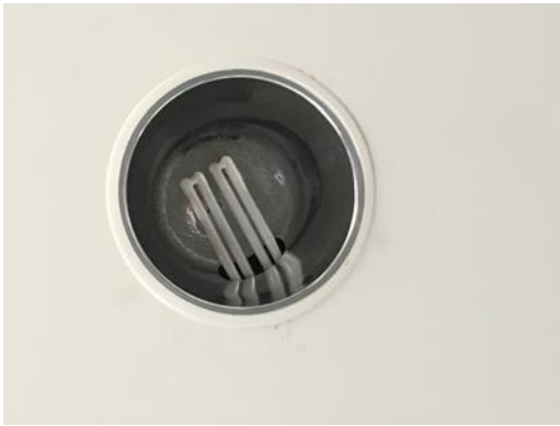
Typical Recessed Can Fixture with CFL Plug in Lamps
