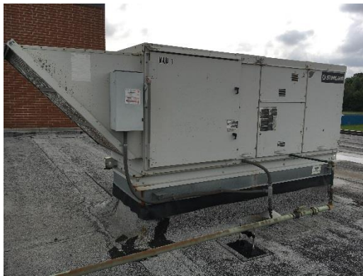
Gas Fired Make Up Air Unit
