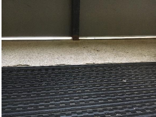
Exterior Door with No Weather-Stripping
