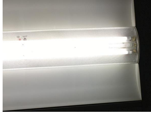
Cafeteria 4-foot 3-lamp T5 Indirect Fixture
