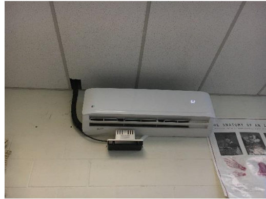
Split AC Systems – Indoor Unit
