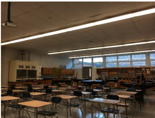
Classroom with 4-foot 2-lamp T8 Wrap Fixtures
