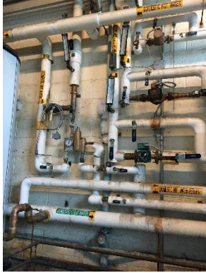
Domestic Water Piping and Circulation Pumps
