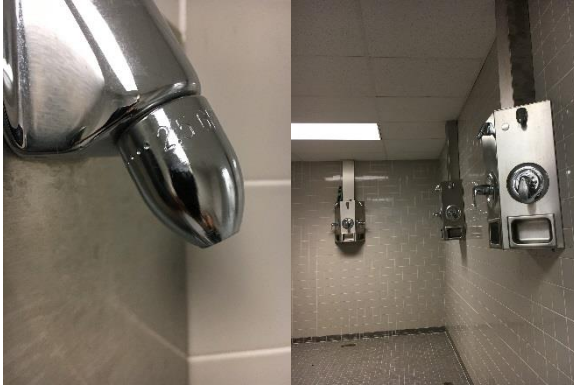
Locker Room High Flow Showerheads
