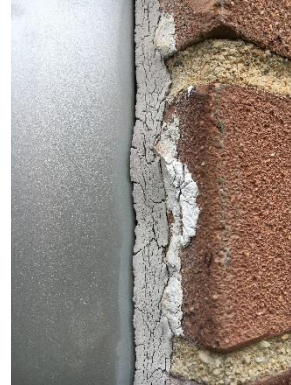
Exterior Wall Frame Caulk in Poor Condition
