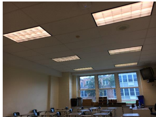
Classroom with 4-foot 3-lamp T8 Troffer Fixtures
