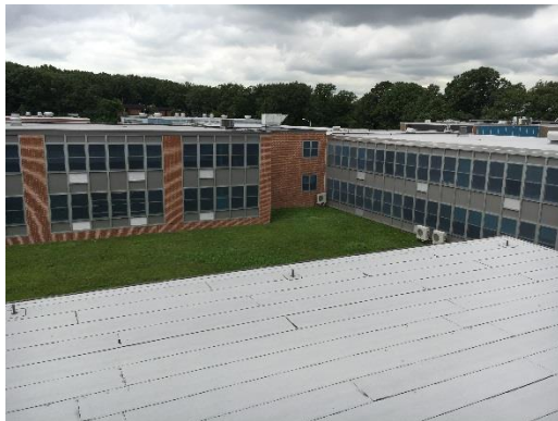
Building Façade and Roof
