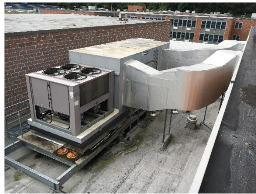
Energy Recovery Unit (ERU)
