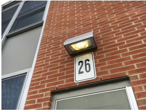
Typical Wall Pack Fixture – On during Daytime
