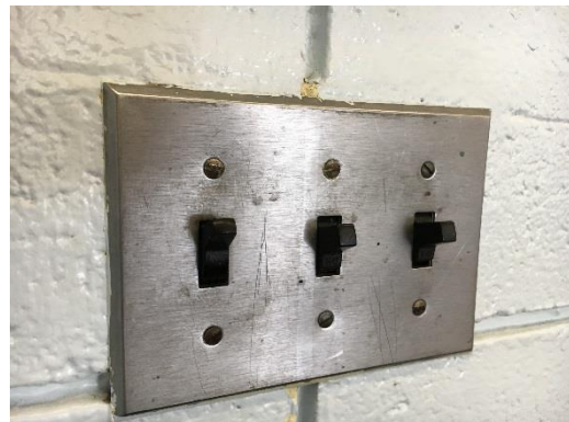
Interior Wall Switches
