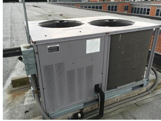
Split AC Systems – Outdoor Condensing Unit
