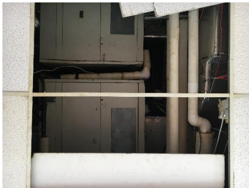
Ceiling Unit Heaters (CUH)
