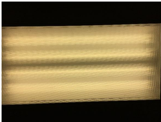
Typical 4-foot 4-lamp T8 Fixture
