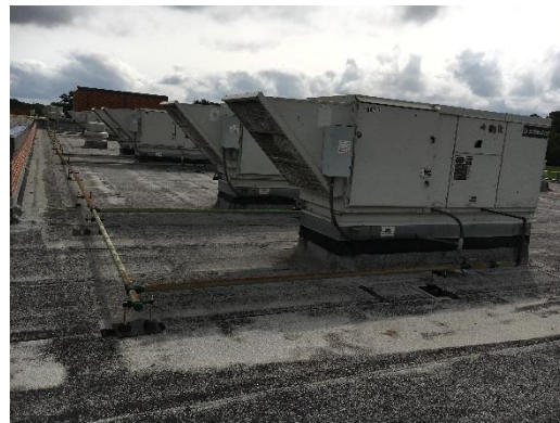
Gas Fired Make Up Air Units
