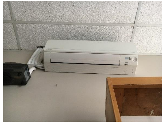
Split Heat Pump Systems – Indoor Unit
