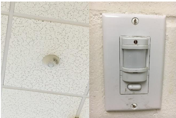
Interior Occupancy Based Sensors
