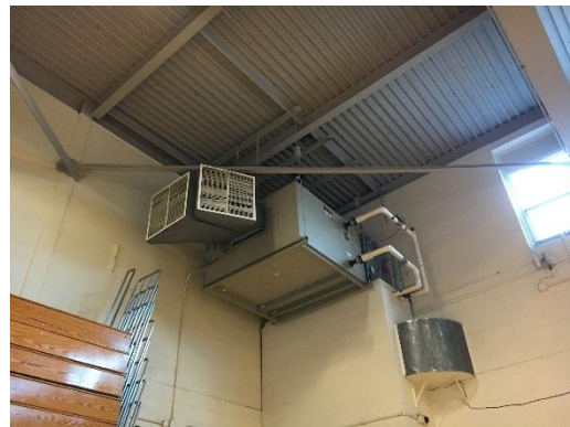
Heating-Ventilation (HV) Unit
