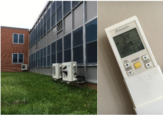
Split Heat Pump Systems – Outdoor Condensing Units
