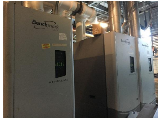
Condensing Hot Water Boilers
