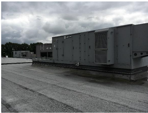
Energy Recovery Unit (ERU)
