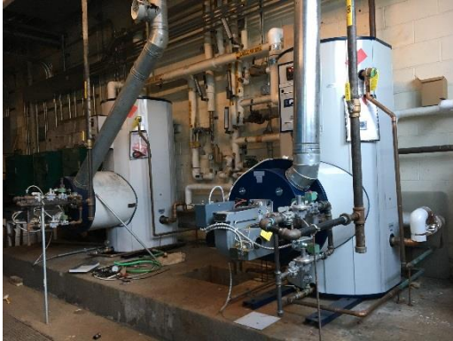
Main Storage Tank Water Heaters
