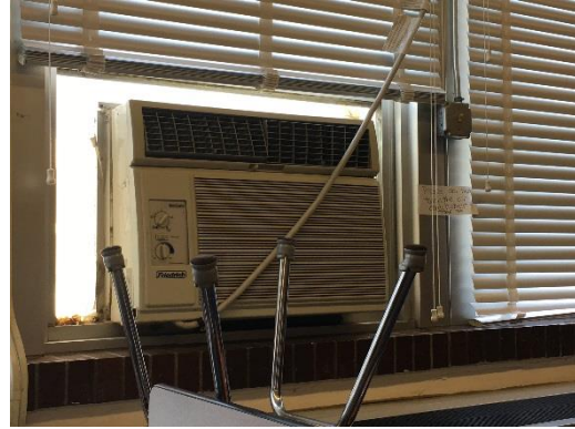
Older window AC unit
