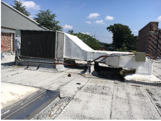
Packaged roof top unit (RTU)
