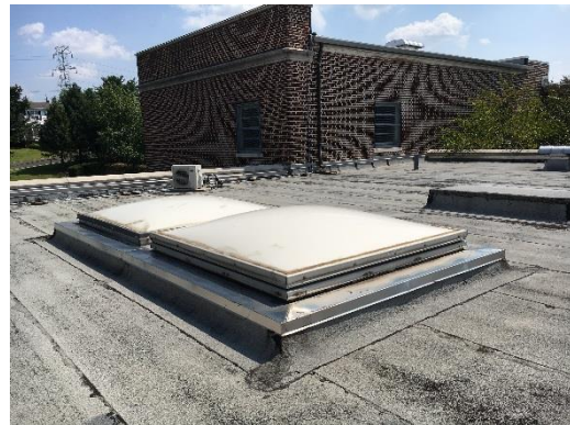
Roof and skylights
