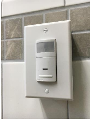
Wall switch occupancy sensor in recently renovated restroom
