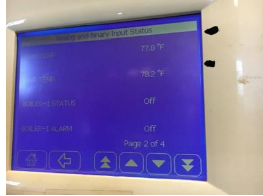
Trane heating controls in Boiler Room
