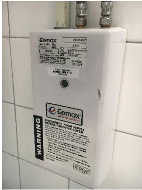
Typical electric tank-less water heater located in recently renovated restrooms
