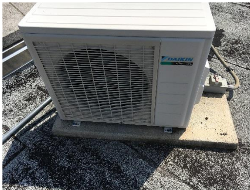
Split AC system – outdoor condensing unit
