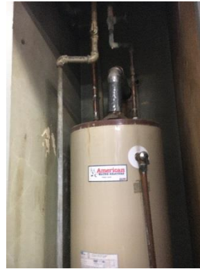
Gas-fired storage tank water heater with no pipe insulation
