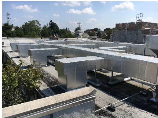
Packaged roof top unit (RTU)
