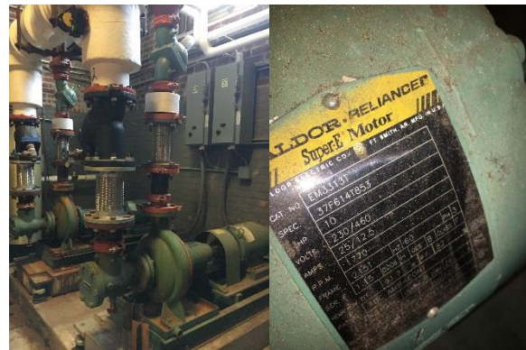
Hot water pumps and motors
