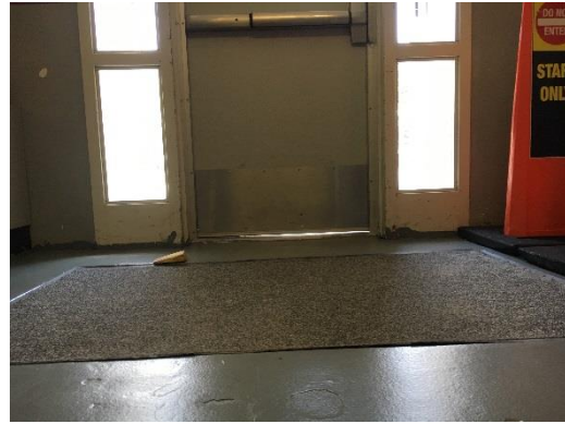
Exterior door with no weather-stripping
