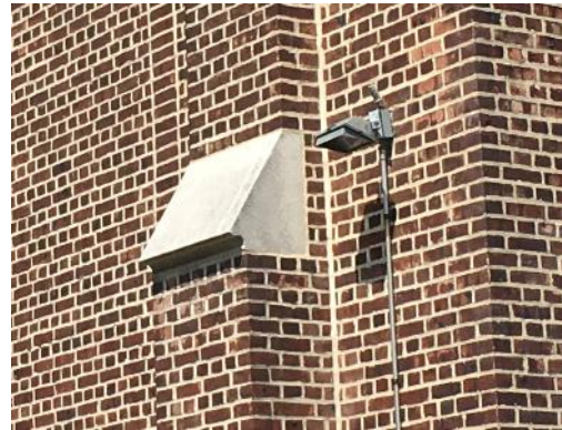
Flood Fixture with Photocell Sensor
