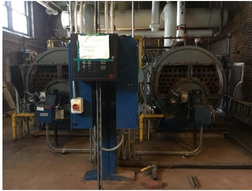
Space heating boilers
