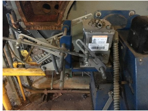
Mechanical linkage burner controls
