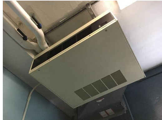
Ceiling Hung Unit Ventilator
