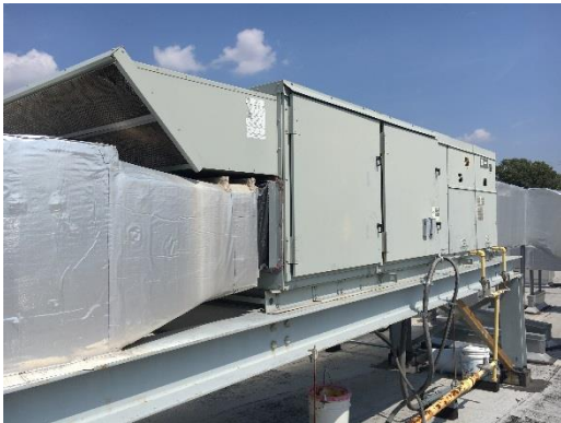
Packaged roof top unit (RTU)
