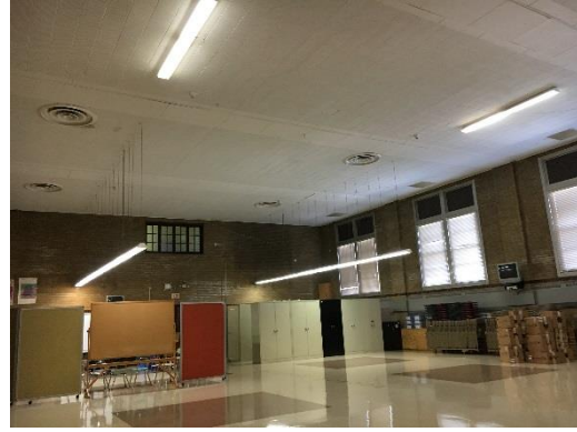
Multipurpose room lighting
