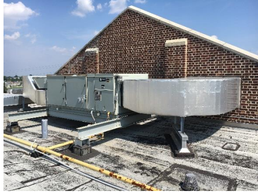
Packaged roof top unit (RTU)
