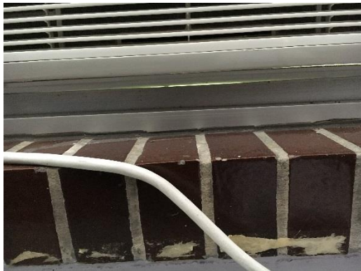
Air gap under AC unit
