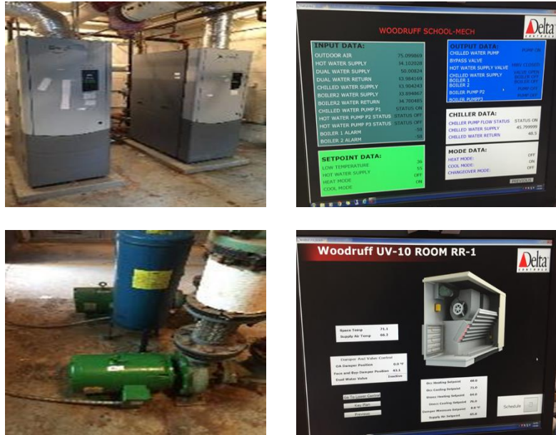
Image 4 Hot water system
