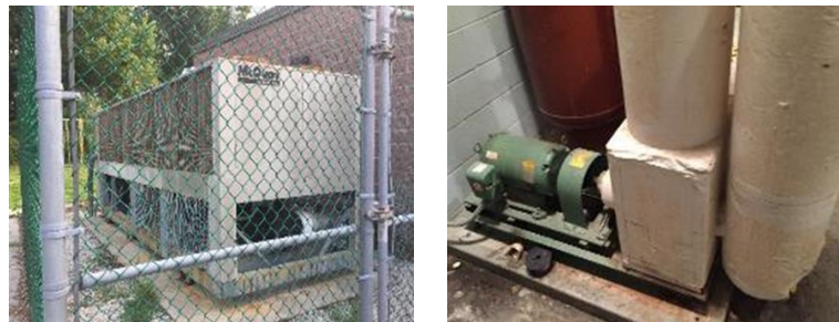
Image 3 Chilled Water System
