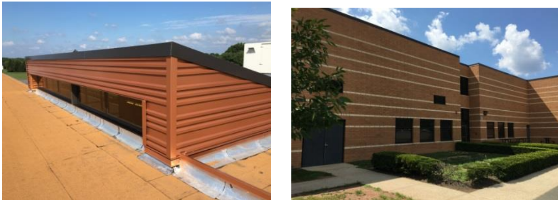
Figure 7 - Building Rooftop and Exterior
