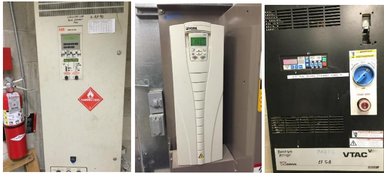
Image 3: All large fan motors are controlled by VFDs
