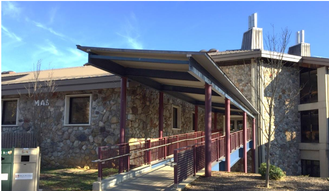
Image 1: MAS Building – Front Exterior
