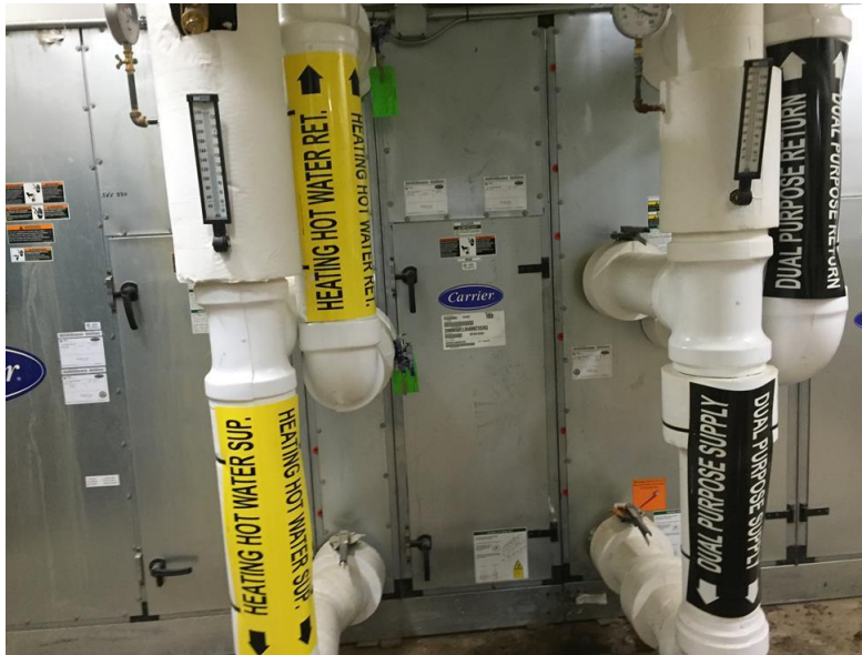
Image 2: Air Handling Units receive hot and chilled water from the Central Plant
