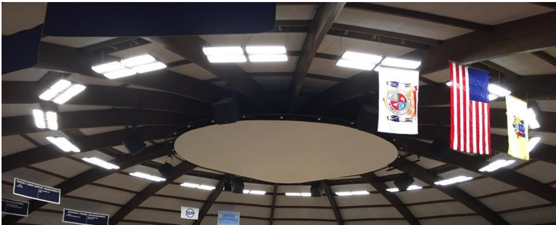
Image 1: Lighting at RCA
