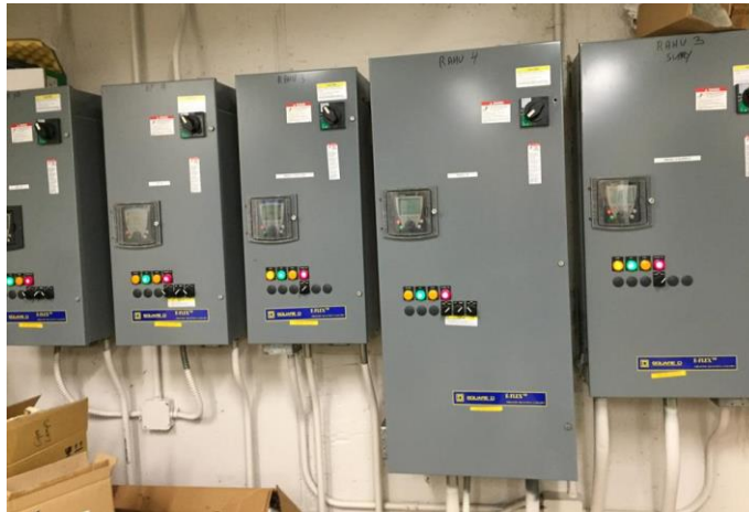
Image 4: All large fan motors in the building are controlled by VFDs
