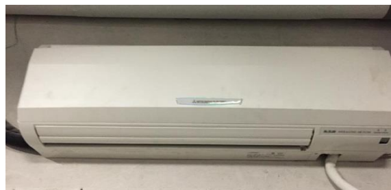
Image 3: Ductless Mini-Split System
