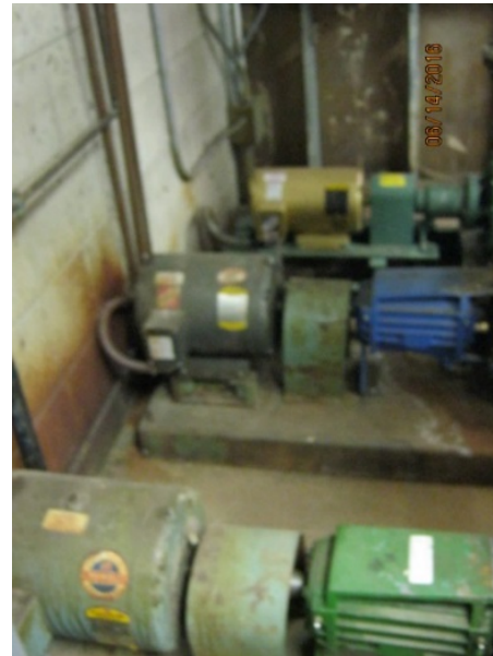
Image 4: Hot Water and Chilled Water Pumps
