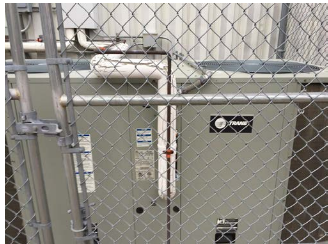
Image 3: Air Cooled Chiller Condensing Unit
