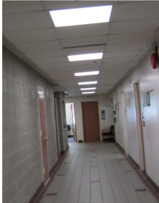
Image 2: Russell Building - Hallway Lighting
